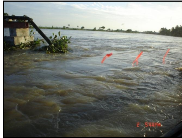
Photo 3: Damaged Road at Kittangi
