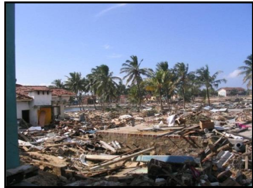
Photo. 4: Damaged Houses at Sainthamaruthu
