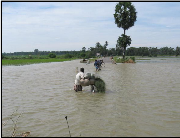
Photo 2: Damaged Road at Kittangi
